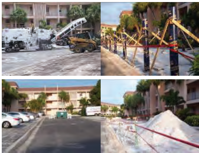
Here is what it looked like during construction.
